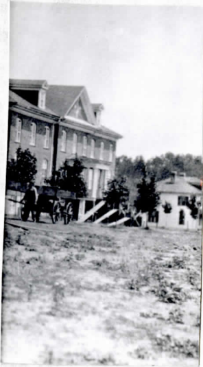
Work on the Campus
